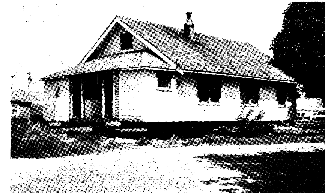
OUT FOR PROGRESS-Old landmark is moved to new location for insurance, real estate and accounting office building and parking area.
